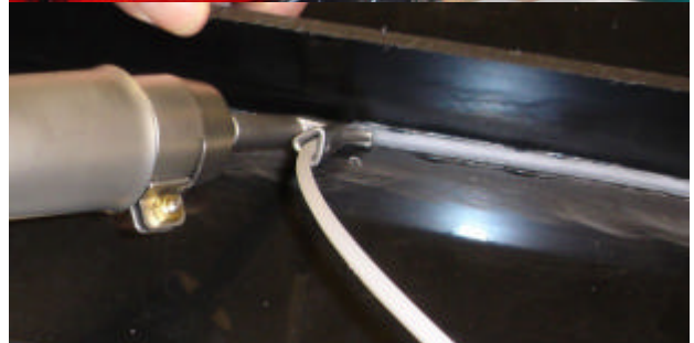
Welding using Speed nozzle
